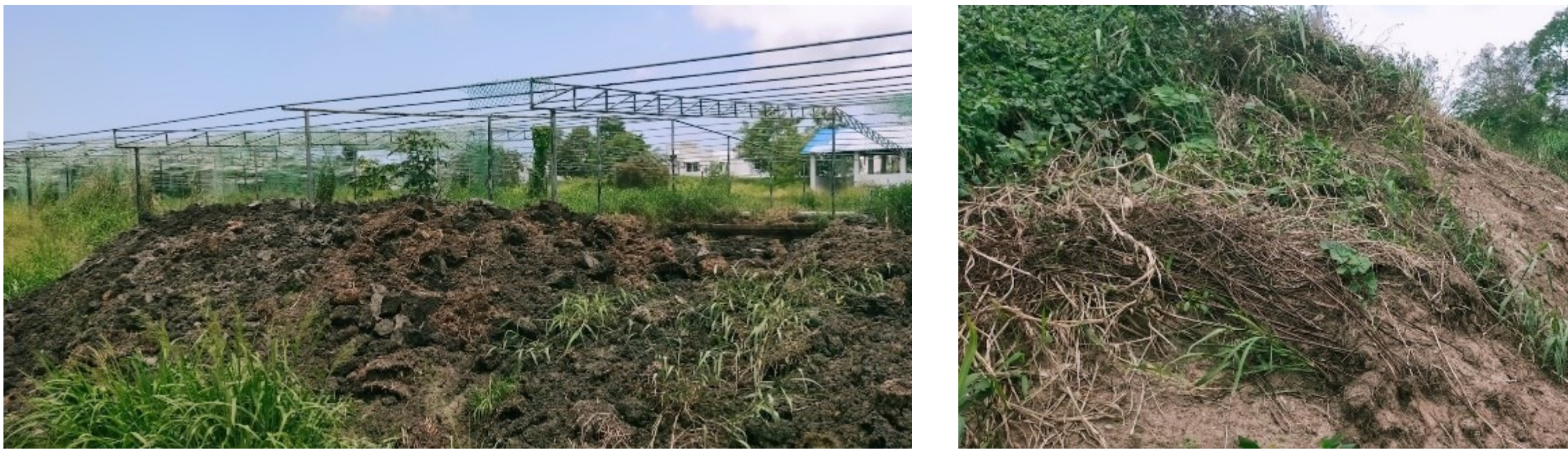
Sludge Buildup in the STP premises
